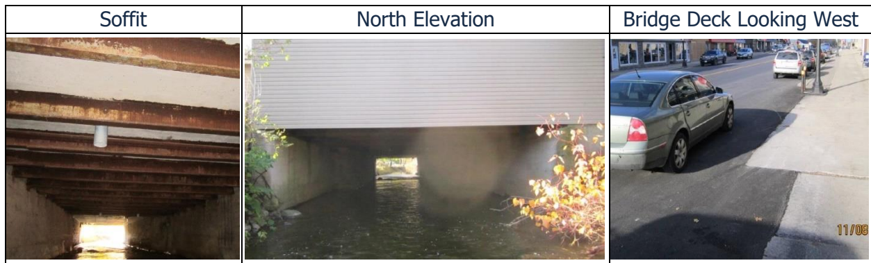
Figure 6: Bridge in Poor Condition (45 BCI)
